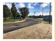
Vierbicher provided professional surveying and engineering services to the City of Dodgeville for their 2021 Street Reconstruction, which included the reconstruction of Leffler and Dydno Street (950 LF), Jewett and Short Street (1000 LF), and Quarry and Dacotah Street (1100 LF), including grading, storm sewer, sanitary sewer, water main, base course, curb and gutter, asphalt pavement, concrete sidewalk, landscaping, restoration of the work area, and other miscellaneous items.
